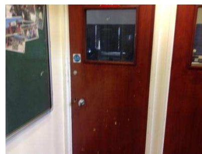
Figure 8. Outside media classroom
